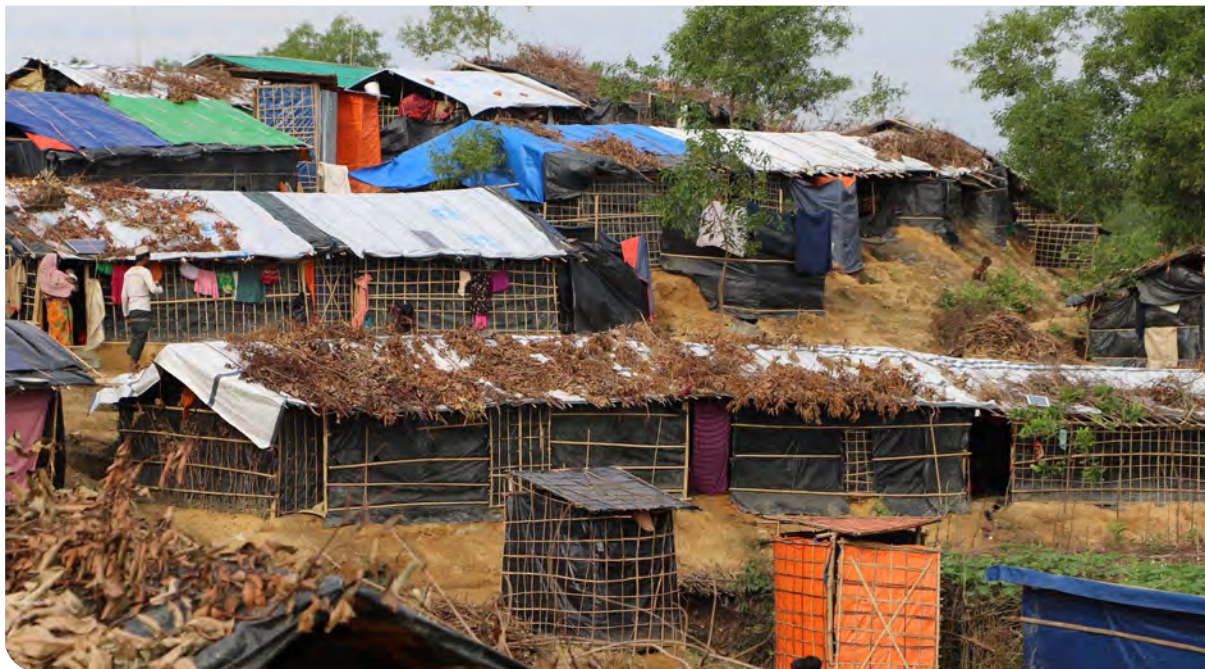
Precarious new settlements in a Bangladesh refugee camp put residents at almost constant risk of landslides and flooding, November 2017
